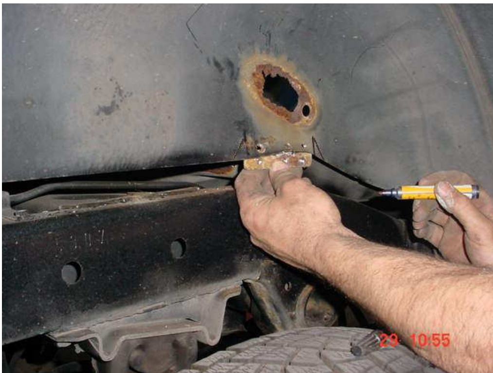
Using the cutoff ends as templates, mark the shape to cut out of the wheel arch lip, to bring it flush with the floor.
