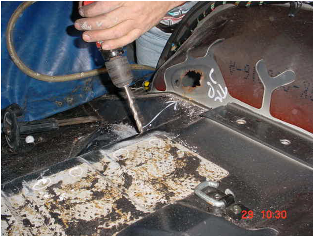
Drill each spot-weld with an 8 mm drill bit (5/16") through the floor only (1 layer). The holes are now prepared and ready for later plug-welding.
