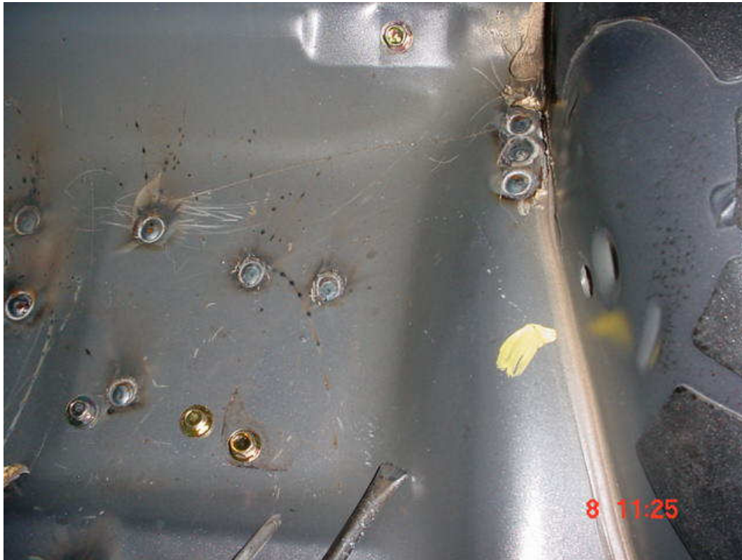
Plug-welds in the central floor area have been welded, ready to grind flush.
