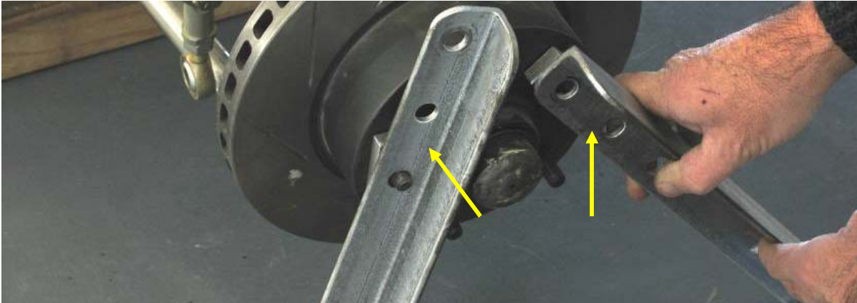
Image 16 - Installation of the bars. The bars can be fitted on to the studs with any of the three holes in each bar.
